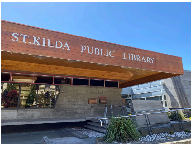
2024, south elevation to Carlisle Street. The original building is to the left with the 1990s addition visible in the background.
