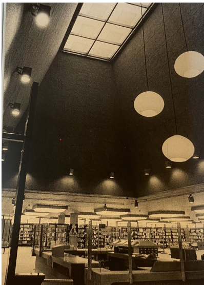
1973, interior, entrance. Source: The Contribution of Enrico Taglietti to Canberra's Architecture.
