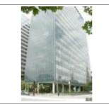
ICI House, Melbourne (VHR H0786), is significant for its considerable advancements in local construction techniques, including framed glazed curtain walls and innovative use of concrete, including precast reinforced units in structural members and flooring. The division of the glazed office space from the solidly clad service tower predates similar developments overseas.
